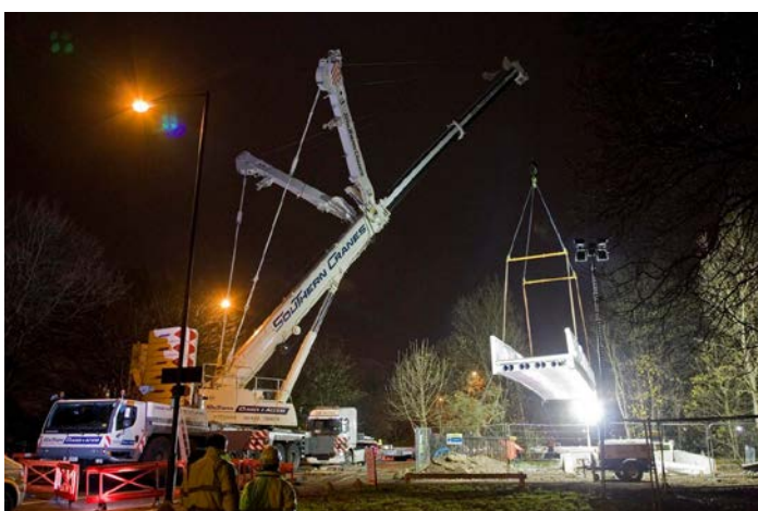
Construction in progress on Lea Bridge Road site
