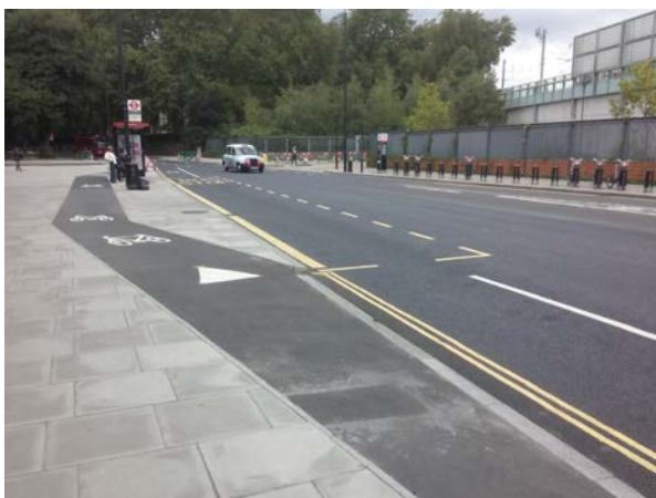
Pancras Road northbound bus stop bypass
