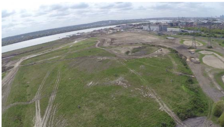
Aerial view of the Barking Riverside development site
