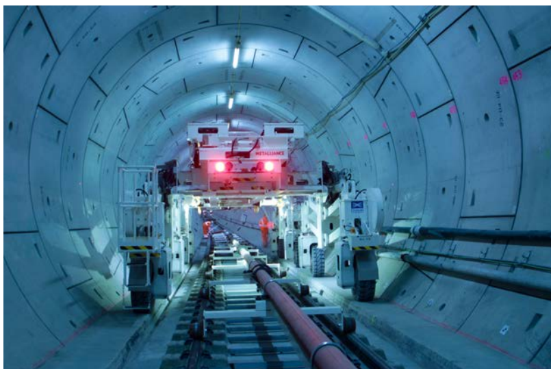
Track laying in Thames Tunnel using a multi-purpose gantry
