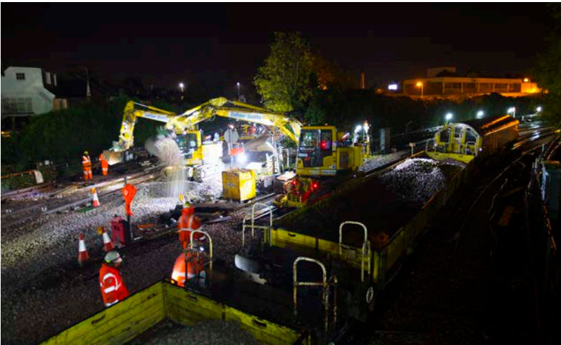
Work in progress at Hanger Lane
