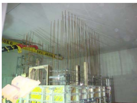
Step-free access lift shaft steelwork
