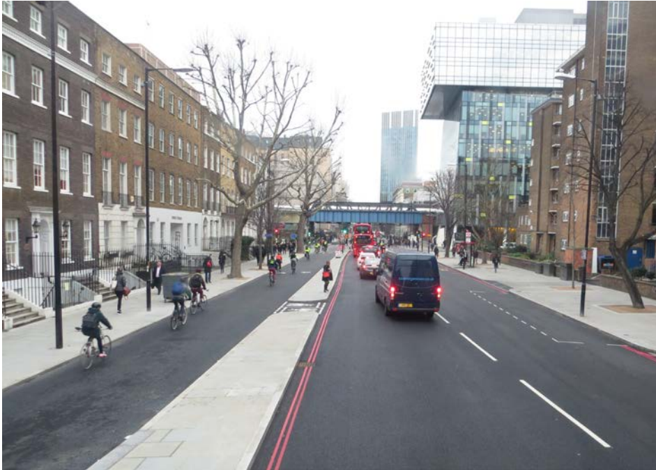
New section of the North-South Cycle Superhighway in use on Blackfriars Road, Southwark
