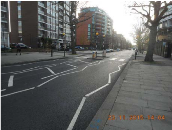
A5205 St John's Wood Road carriageway resurfacing
