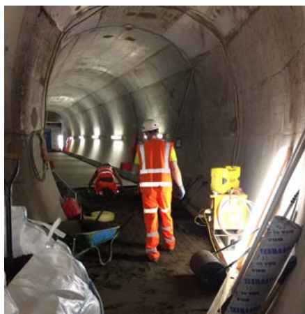
Works in progress within the paid area link
