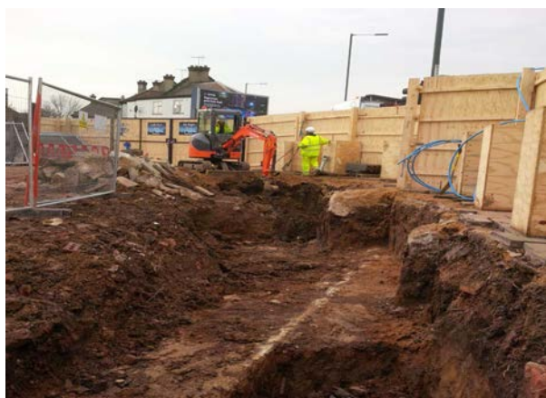
Brentfield Road site excavations
