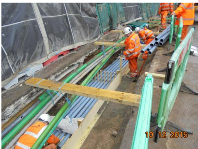
Utility diversions in Arthur Street
