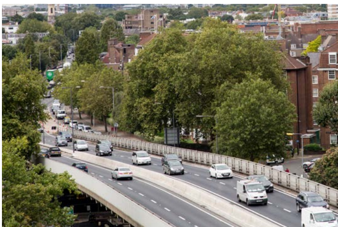
Hammersmith Flyover with its new reinforcement structure
